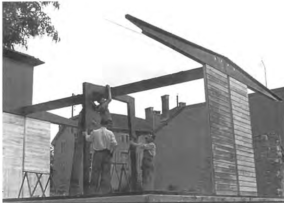
Figure 3. Houses for victims of war, Nancy, 1945. Buildings under construction. (© ADMM)
