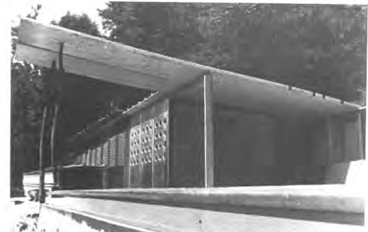
Figure 8. Jean Prouvé's own house, Nancy, 1954. Building under construction. (© Centre Pompidou, Bibliothèque Kandinsky)
