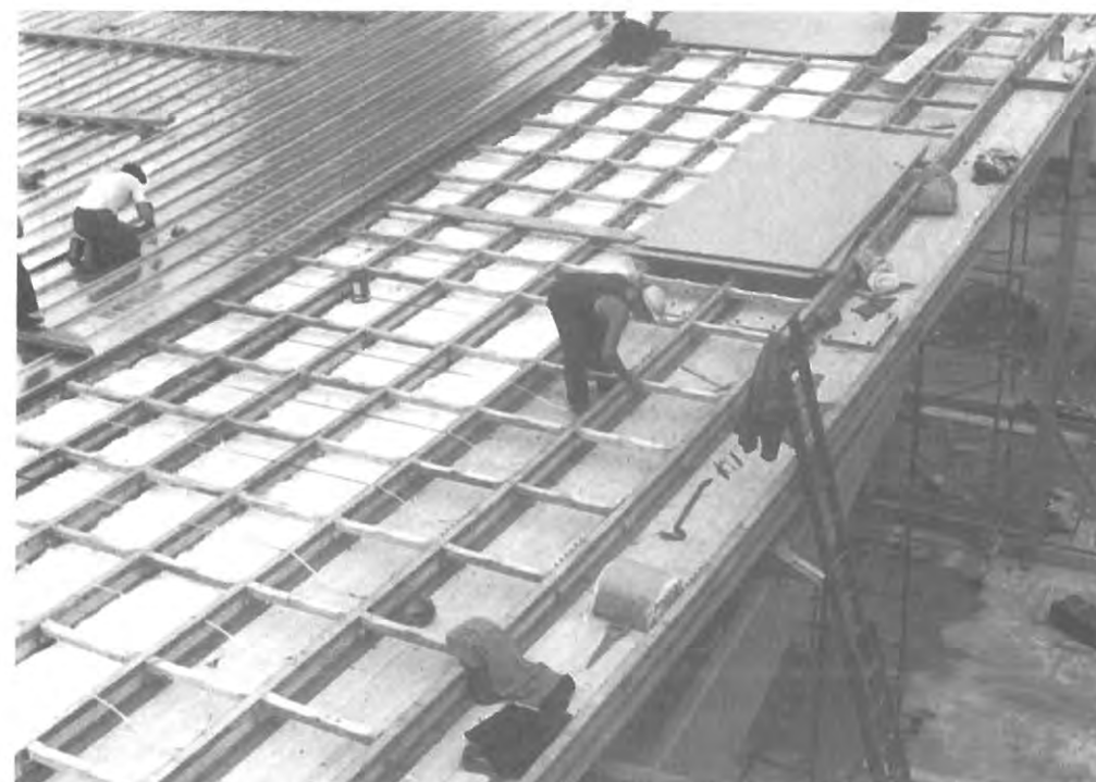
Figure 14. Pump Room, Evian (Haute-Savoie), 1956. Roof under construction. (© Centre Pompidou, Bibliothèque Kandinsky)
